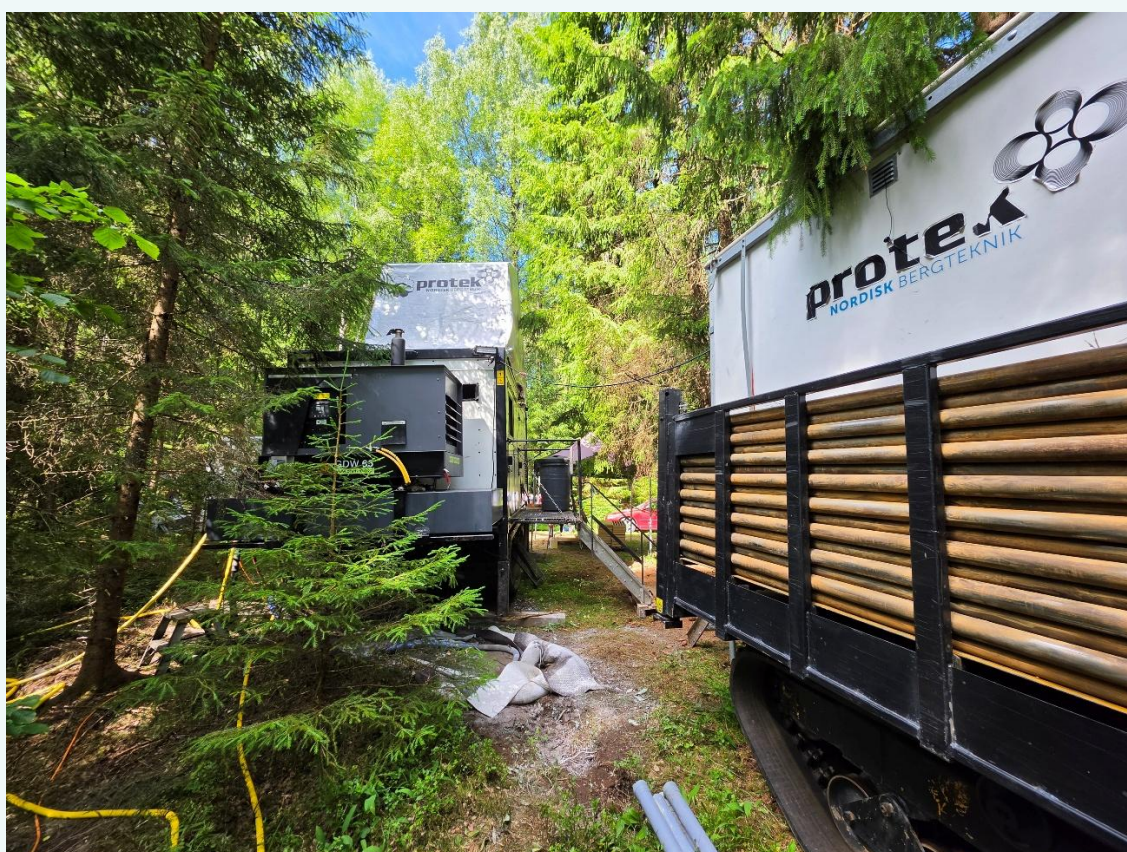
Figure 7. Drill rig in action at the Hennes Bay project
